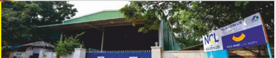
DOORS UNIT: Phase-III, IDA, Jeedimetla, Hyderabad, Telangana - 500 055
